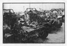
SOCCENT troops take breather next to FAVs (fast attack vehicles) at Kuwait City International Airport. Fast (80 mph), adaptable, FAVs carried 40mm Mk 19 Mod 3 automatic grenade launcher, M60s, "Ma Deuces," M136 (AT4) light antiarmor weapons, TOWs and 30mm ASP-30 cannons. Many driven by SEALs carried M14 in mount by driver.
